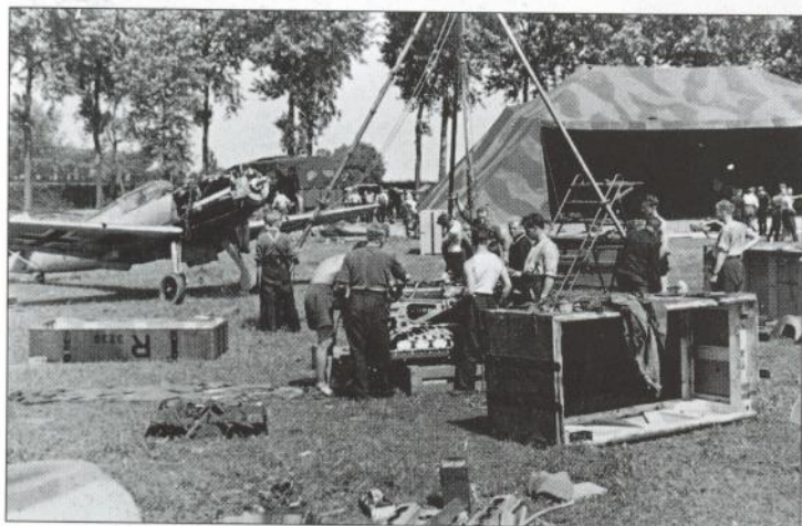
Groundcrew uncrate a replacement DB 601 newly arrived from Germany prior to carrying out an engine change
