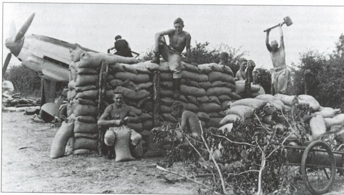
Constructing yet another sandbag blast pen similar to that protecting Schöpfel's machine
